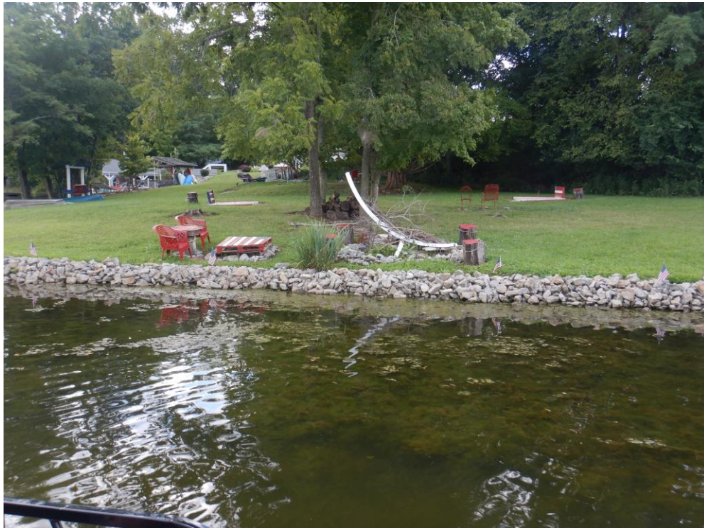
Photograph 6. Additional properties had no natural buffer between mowed lawn and lake.
